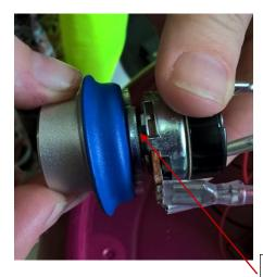
11. Slot the motor through the motor holder so it is poking out, making sure the thick metal washer is between the motor and the motor holder (photo is taken with the parts not slotted into the grill to demonstrate).
